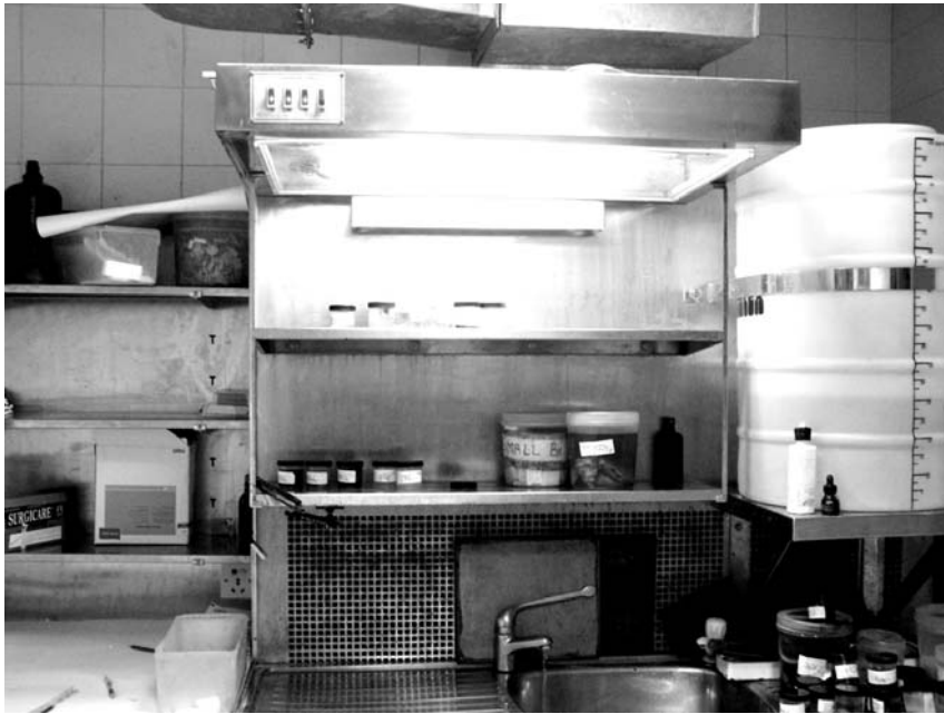
Fume hoods in pathology labs, such as the one above, protect workers from formaldehyde fumes.
